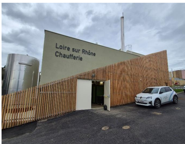
Chaufferie biomasse de Loire-sur-Rhône
